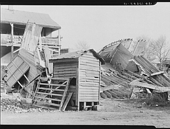
Flood damage. Shawneetown, Illinois
