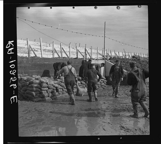
Piling sandbags along the levee during the height of the flood. Cairo, Illinois
